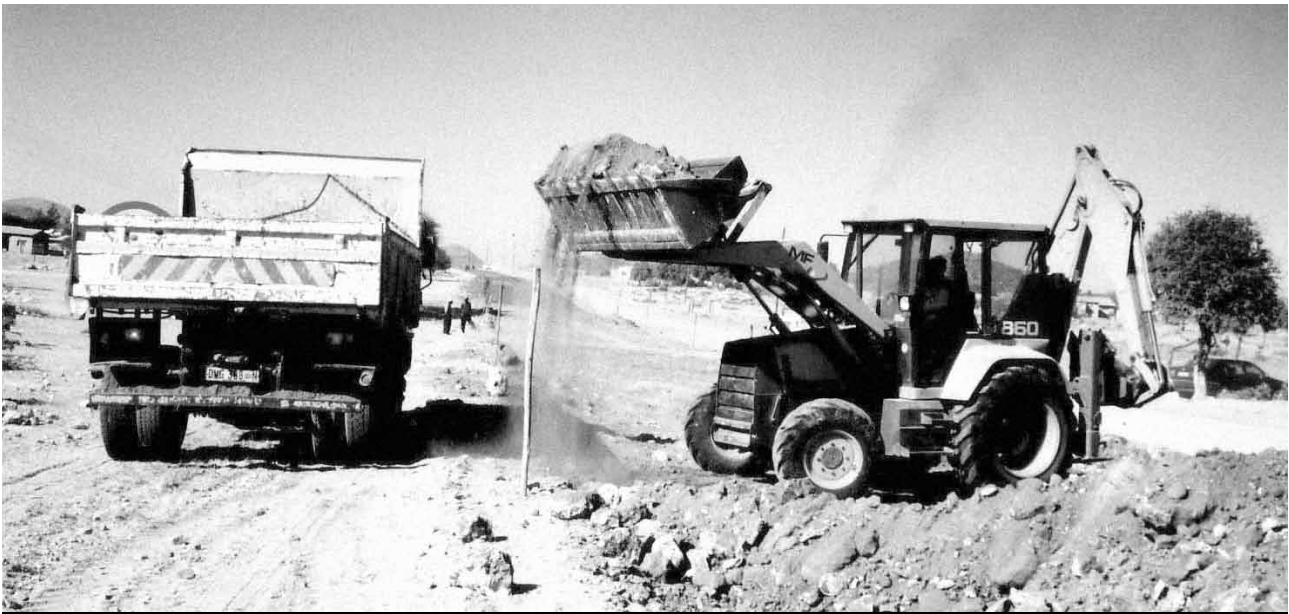
Road construction in Makurung village, Ga-Mphahlele district, Limpopo.
