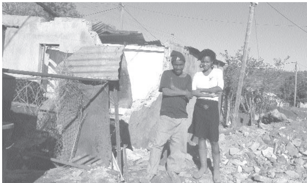
Kholisile Mnika and Nomalanga Mkhize stand on the rubble of a house which fell because residents were told not to build deep foundations because of graves beneath
