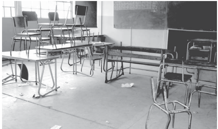
Dromedaris primary school in Reiger Park, East Rand is in a disgraceful condition.
