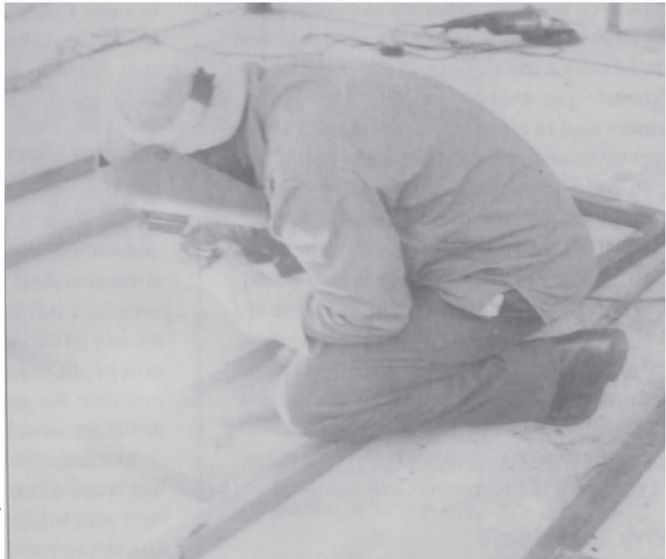
The MDA trains micro entrepreneurs in window frame making at Mhala in the Northern Province.
