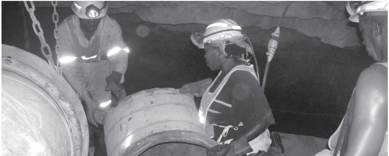
An underground woman worker carrying a ventilation pipe.
