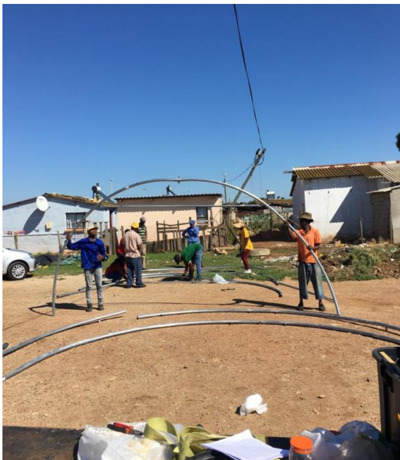
Saltuba co-op members erecting a food tunnel on the gap tap
